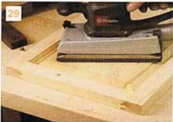
29 A light sanding once dry will flush off the joints
