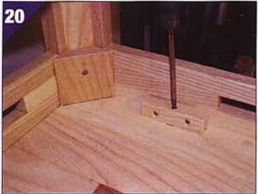
Carefully lift the leg and rail assembly onto the underside of the table top, and align. Fix with screws through the attaching blocks
