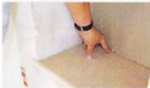
▲ Pic. 5 Once you cut to this line, the result should be a board that drops into the opening for a perfect fit on all edges
