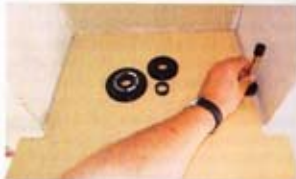
▲ Pic. 1 A loose fitting template is dropped into place and a suitably sized wheel is pushed against the walls and run around them to make an offset mark
