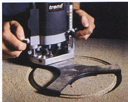
Simply rout a circle to create an access hole
