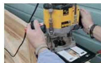
A heavy-duty router is needed to rout out the lock case, or you can drill and chisel if needed
