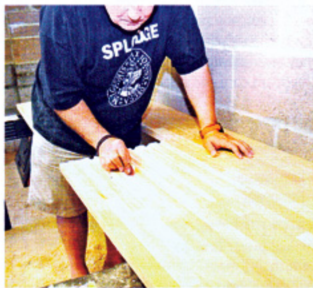
▲ A bit of light sanding and it's ready for fitting and finishing
