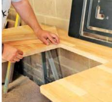
quite heavy and although still clamped to the jig during the cutting process, will still prove a dead weight once it becomes free of the worktop. This can, as I found, twist the jig slightly, making the cutter dig marginally into the newly cut aperture. Nothing too drastic though, and easily sorted with a few rubs of abrasive to feather it out.
