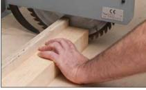
Components are cut to length to suit the aperture size.
