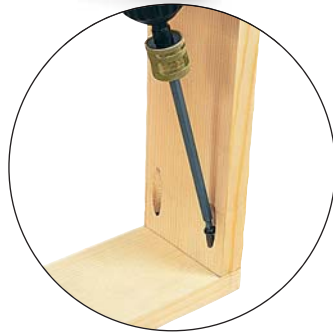
4. Drive self tapping screws to secure.
