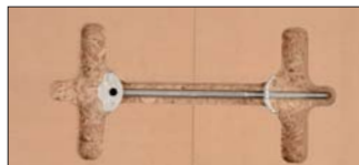
Bolt fitted into recess.
