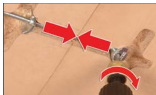
Turn hex bit to tighten Zipbolt and to tighten joint.
