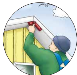
Position the tool in the unknown angle and the metal flag automatically halves the angle.
