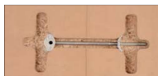
Bolt fitted into recess.
