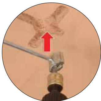
Fit Zipbolt to hex ratchet bit in ratchet screwdriver or torque screwdriver drill and place in worktop recess.
