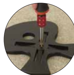
Setting-up The diameter of the finished access hole will be 108mm. Carefully mark the centre point of the circle, if possible positioning the access hatch between the floor joists. Screw the Routabout jig to the floor using a single No.8 particle board screw at the centre point to act as a pivot.
