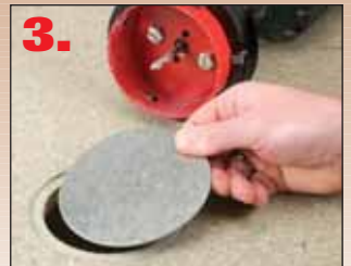
3. Place steel cover plate inside rebate
