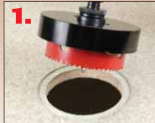
1. Drill into flooring board
