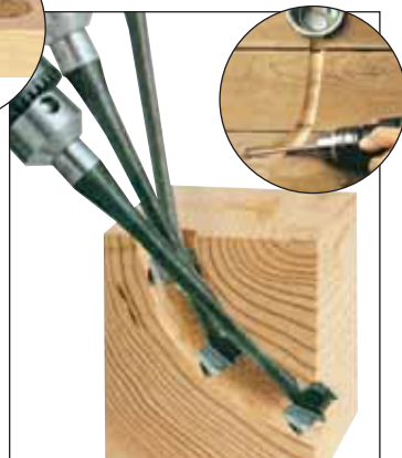
Drill Curved Holes and Cable Channels
