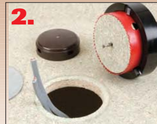
2. Remove waste piece from hole saw and install/retrieve cable
