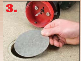
3. Place steel cover plate inside rebate
