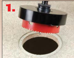
1. Drill into flooring board
