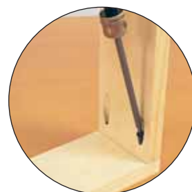
4. Drive self tapping screws to secure.
