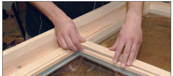
Fit the glazing and beads.
