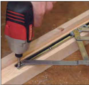
Fit the stays against the datum point for speed and accuracy. The system caters for Friction Stays with 13mm stack height and 16mm base plate.
