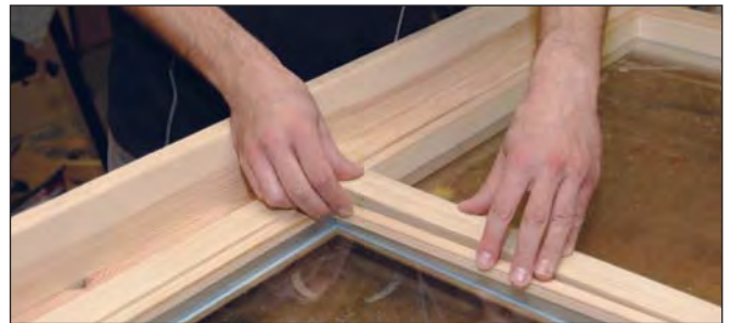
Fit the glazing and beads.
